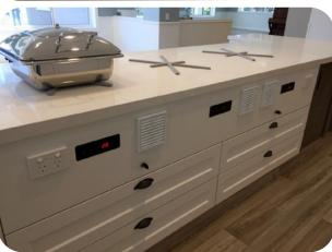
Our French partner ADVENTYS have developed Induc-Stone, a technology that allows chafing dishes to be kept warm with induction units placed under stone benches with single degree temperature precision.
